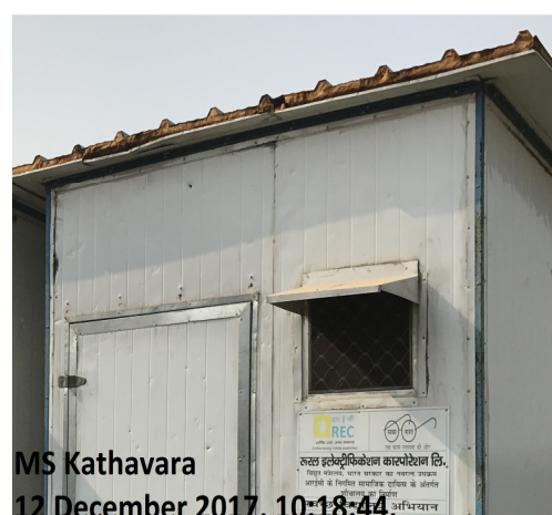
Roof actually constructed
