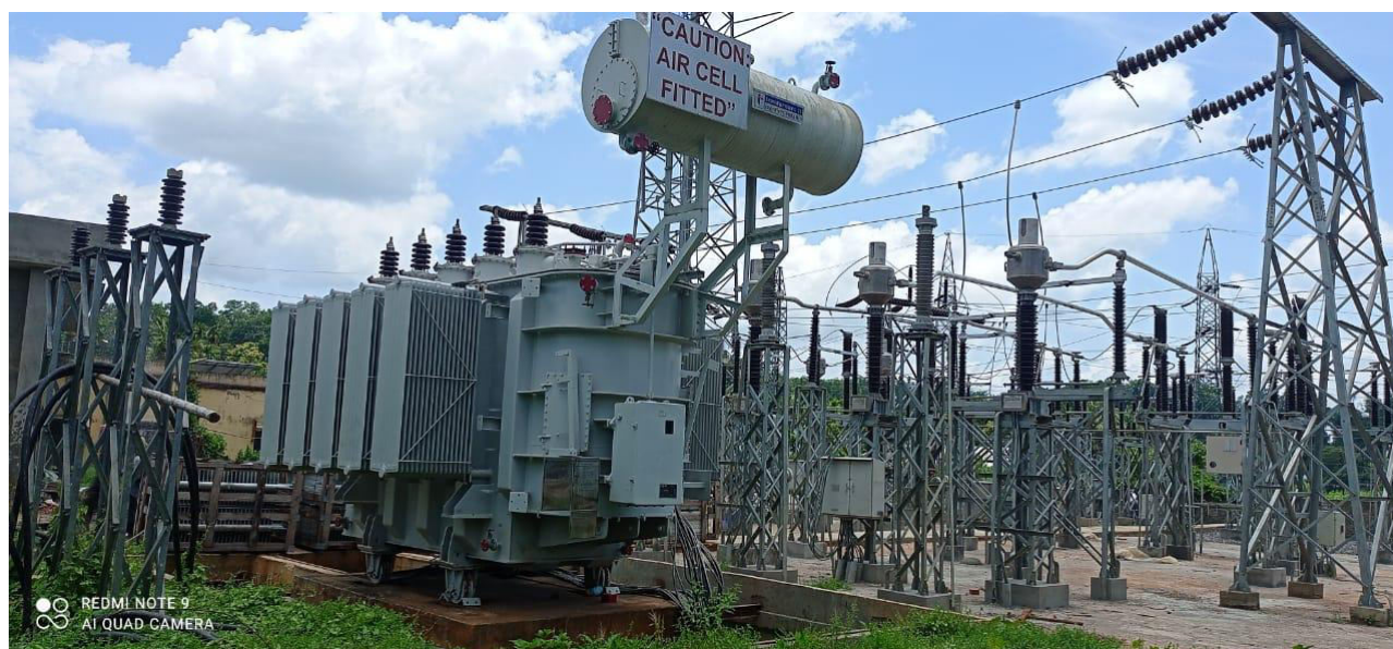
Transformer Erection with Oil pit in Progress – Ambassa S/S
