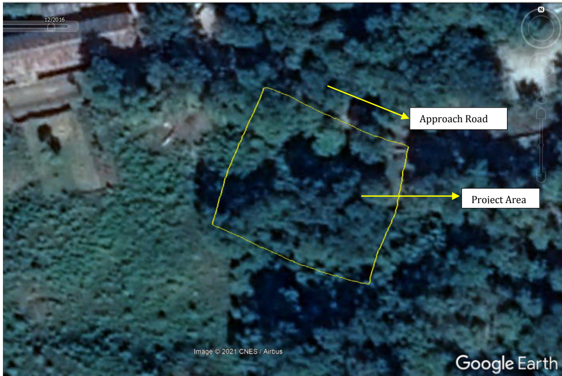
S/S Site in 2017 – Before Construction Work Start
