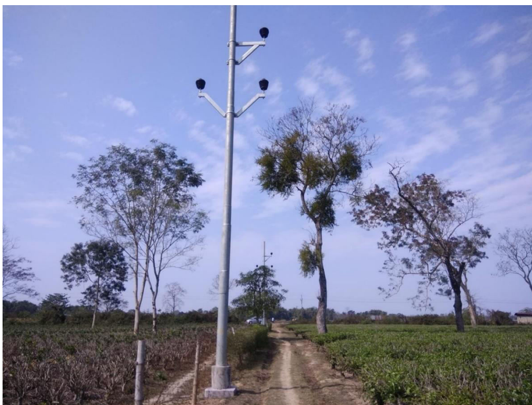
Figure 5-7: Example of Pole erection where Tree is Prevented from Cutting
