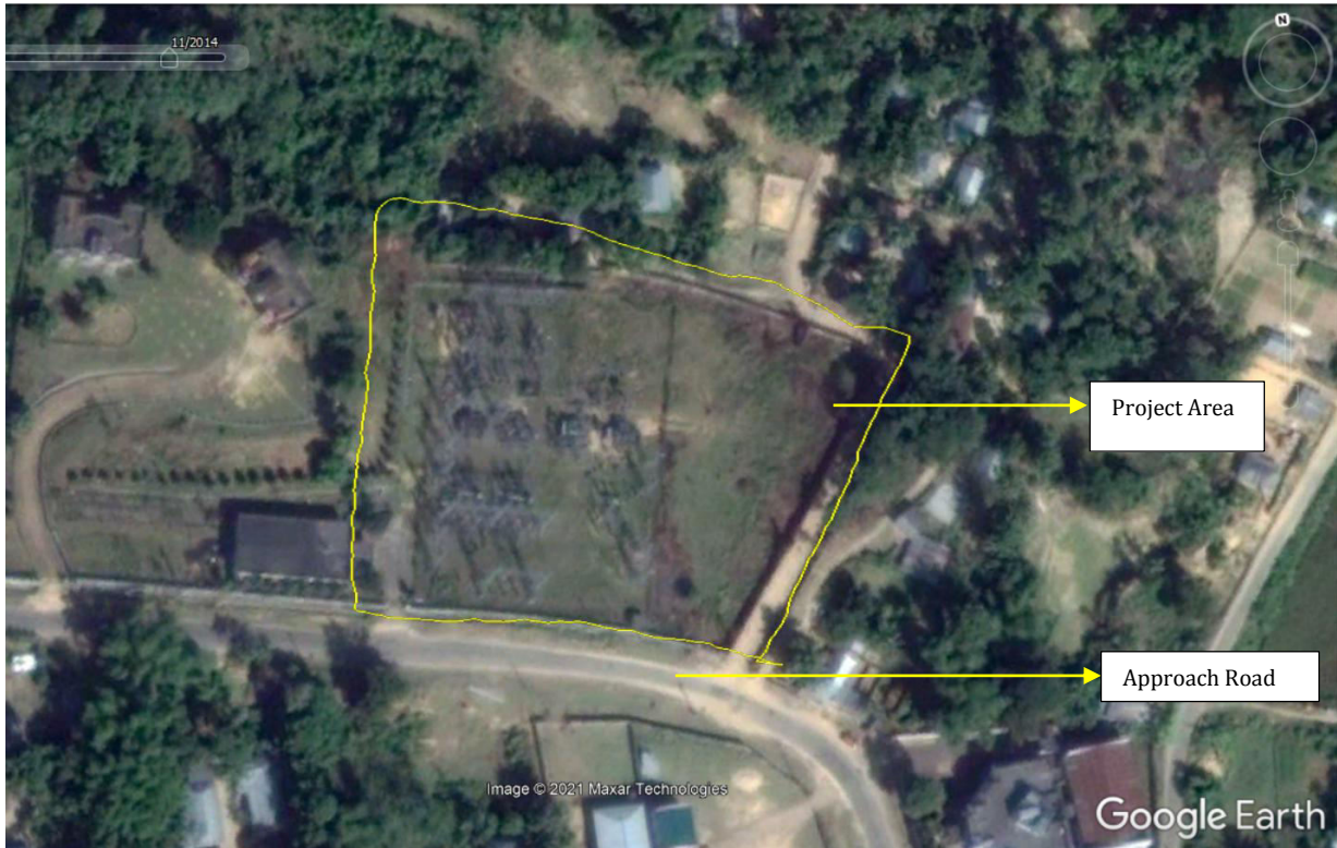
Before extension work - 2017
