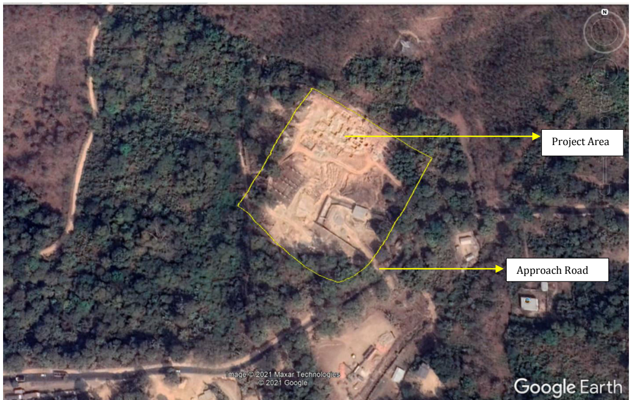
S/S Site in 2021 – Construction Work in Progress
