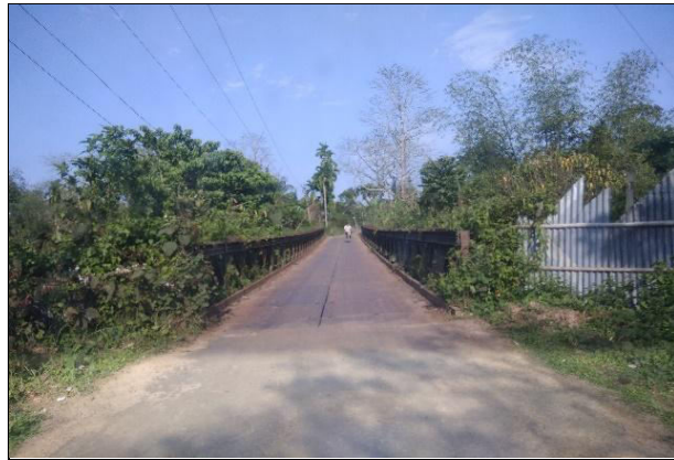
TL Crossing Raiway Line and Bridge
