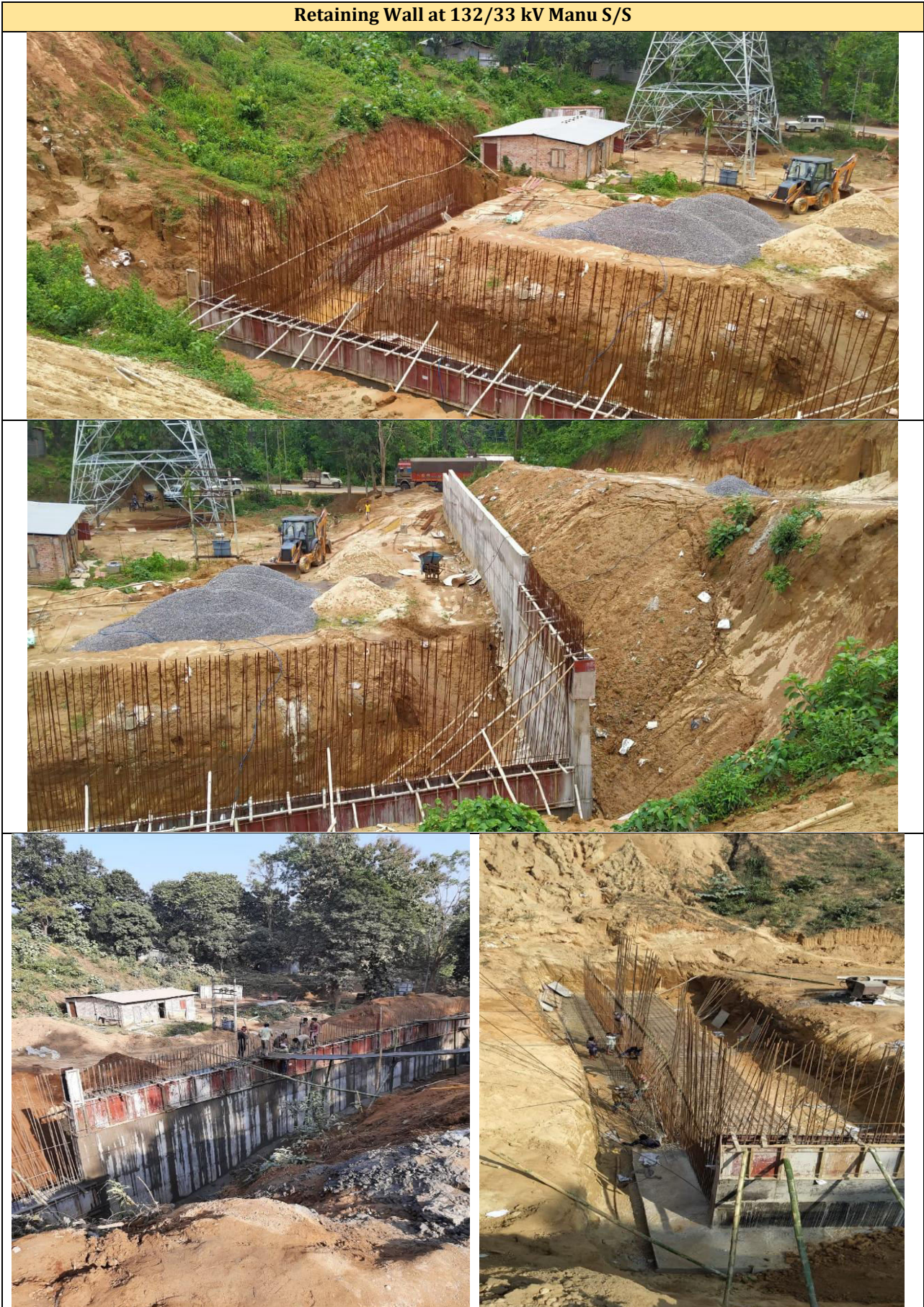
Figure 5-8: Erosion Control Measures
