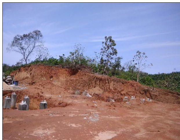
Jawahar Nagar S/S construction site
