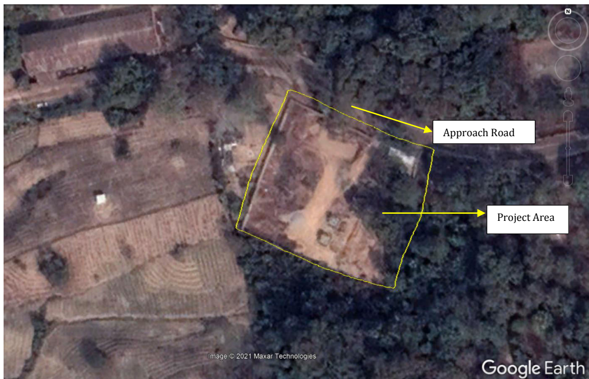
S/S Site in 2021 – Construction Work in Progress
