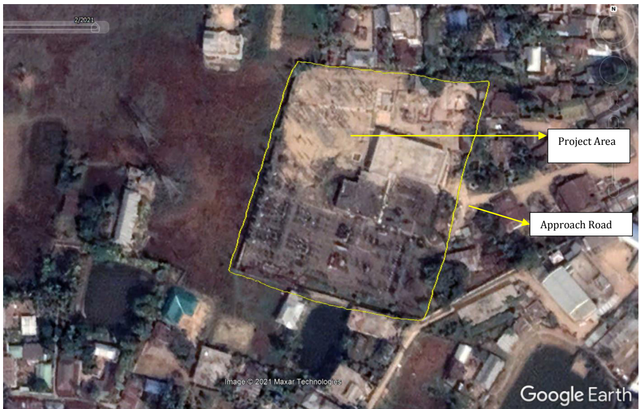
S/S Site in 2021 – Augmentation Work is Completed
