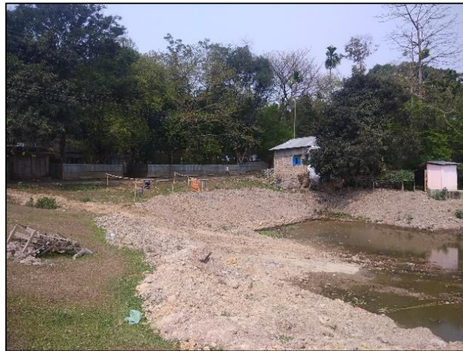
82-mile S/S Construction Site
