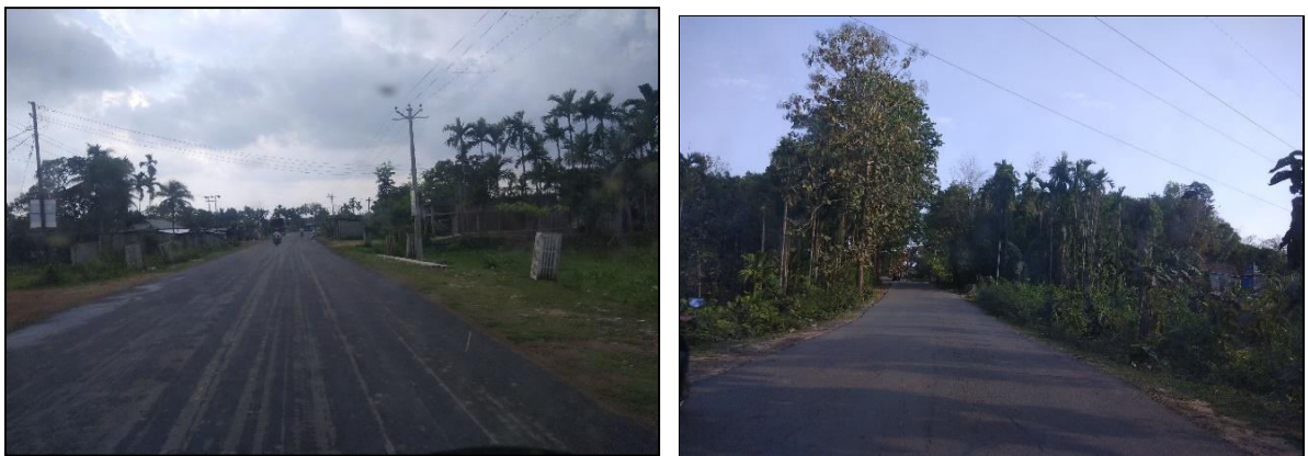
TL Crossing Metal Road
