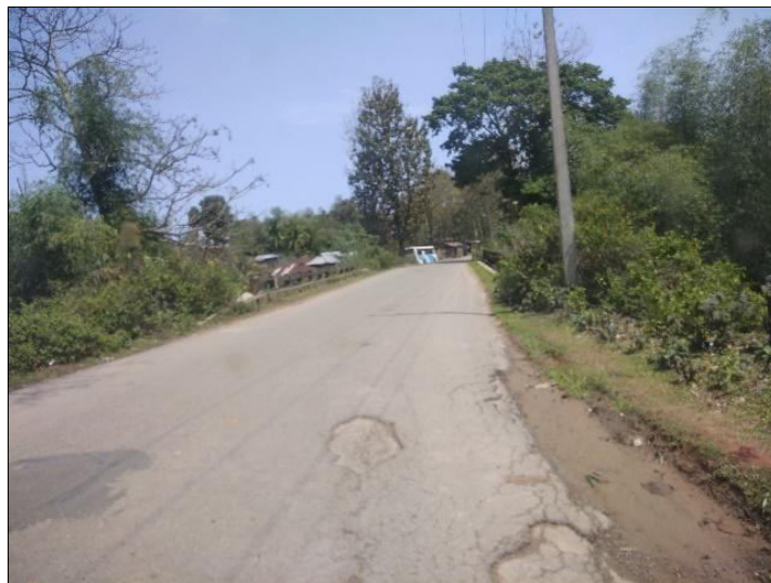
Pole Location along Metal Road
