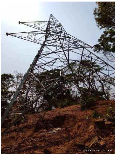
Extension foundation – 132kV Lungsen-Chawgte T/L
