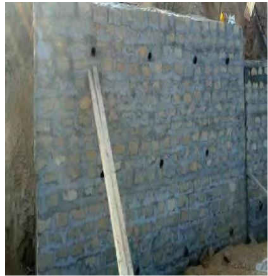
Wall under construction at 33/11 kV South Bungflang S/S
