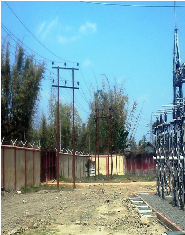
istrict, 33 kV (H Pole) line inside substation
